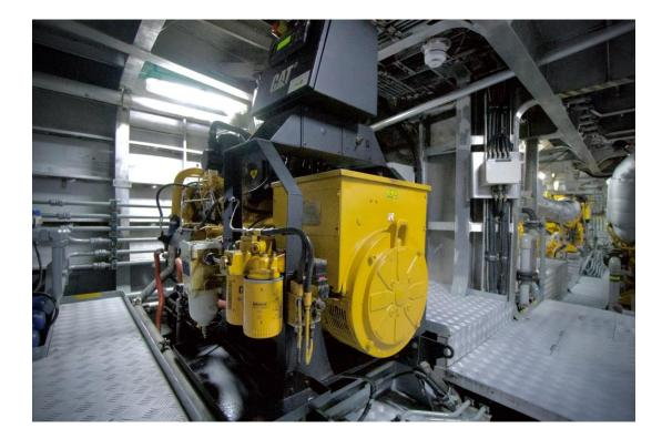
Two generator sets Caterpillar, type C4.4 T, 73.0 kVA 415V/ 240V, 60 Hz AC
