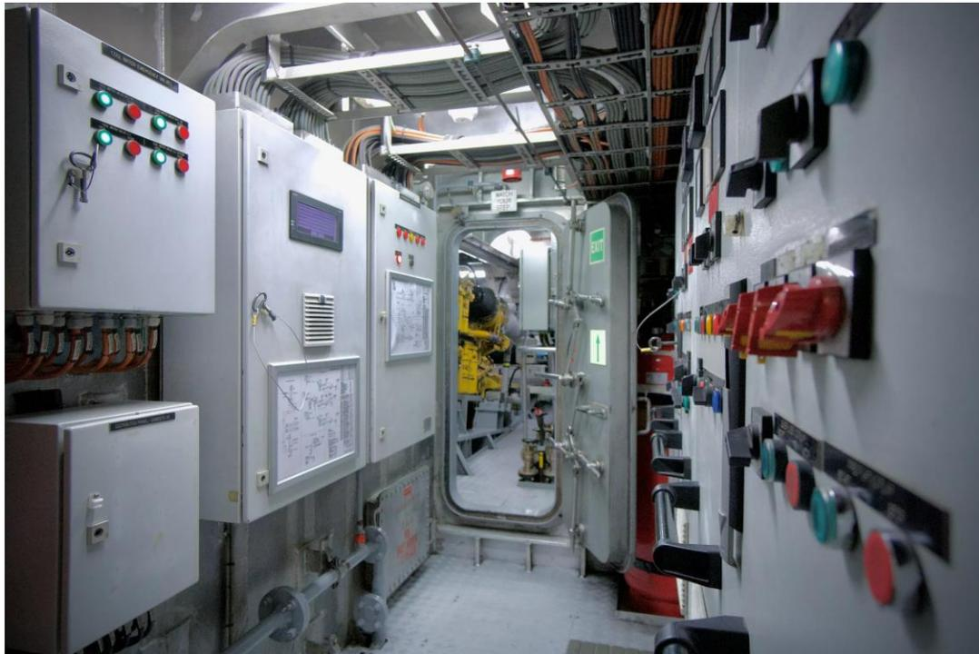
This tank room/control room is separated from the engine room by means of watertight door.
