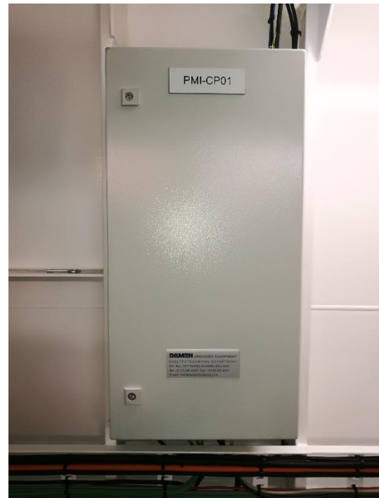
PRODUCTION MEASUREMENT CABIN
